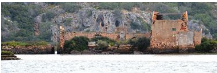
Photo of the remnants of a tidal grinding mill. The guide said it was grinding wheat for flour. You can just see the channel on the left where the wheel would be placed. Why have we forgotten the almost free, natural, renewable resource?
